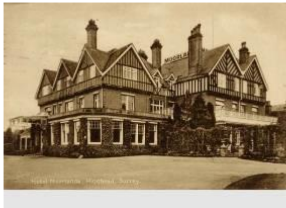
Moorlands Hotel 1890s. Now demolished, turned into the Lloyds Bank Training centre, then British Car Auctions and now overpriced retirement homes
