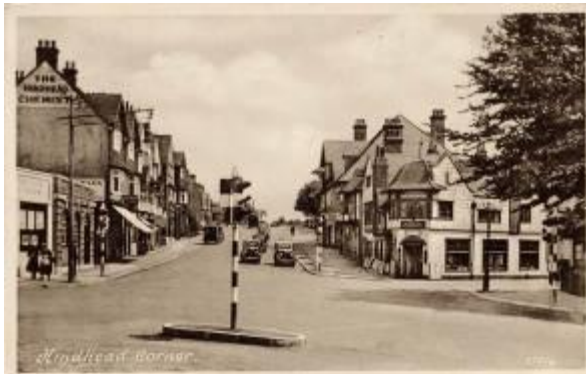
1930s The struggle overpowers the constabulary Traffic lights are installed. Note queue waiting to go South
